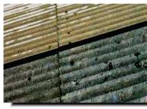
**Figura 7 - Coperture in cemento-amianto**
